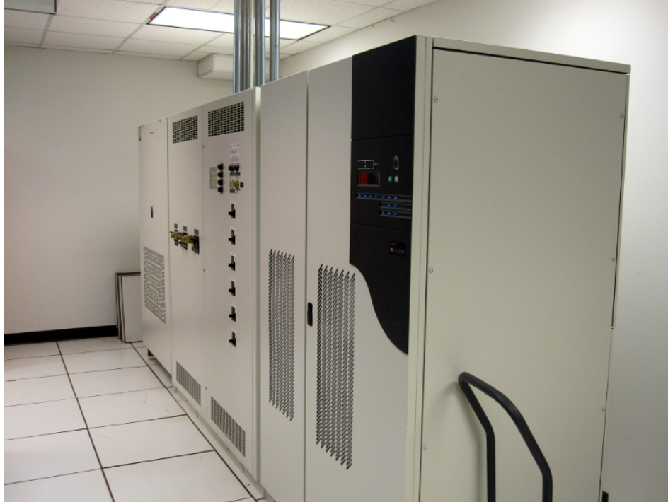
One of two primary UPS's
